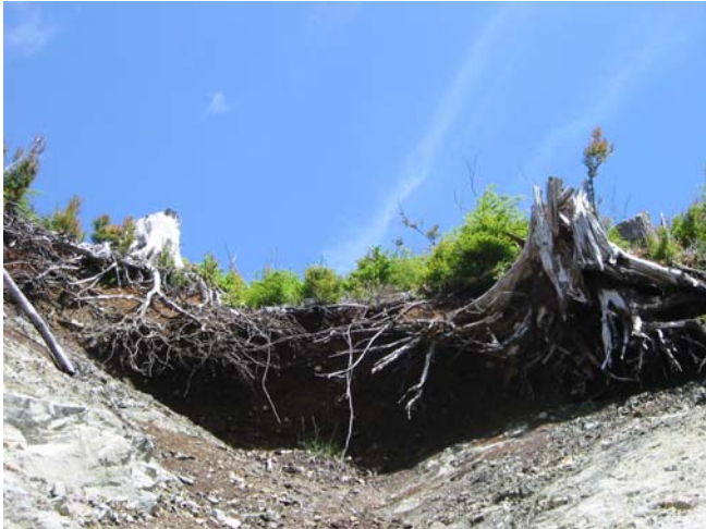
Figure 2 – Landslide headscarp located below two harvested stumps. Headscarp was approximately 1.5 metres high. Slide is located near Bamfield, B.C.
